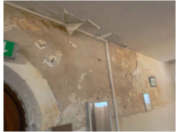
Ceiling and wall of the vestry
