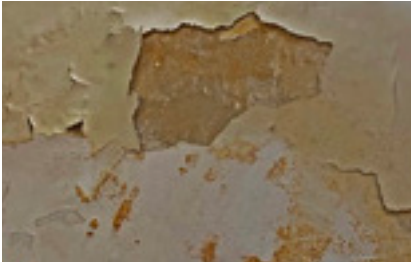
Wall to the right of the altar
